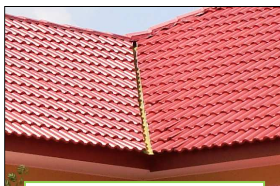
All Main Tiles At The Valleys Must Be Fastened, Nailed, Screwed Properly
