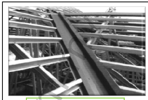
The Gutter Is Installed In The Valley Of The Roof
