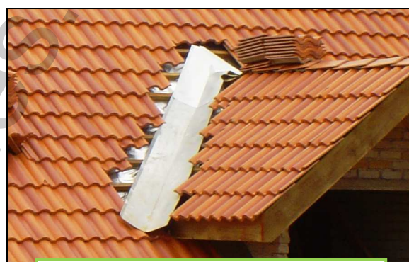
The Main Tiles At The Valleys Must Be Cut To Allow The Correct Valley Gap
