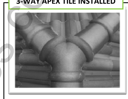
3-WAY APEX TILE INSTALLED
